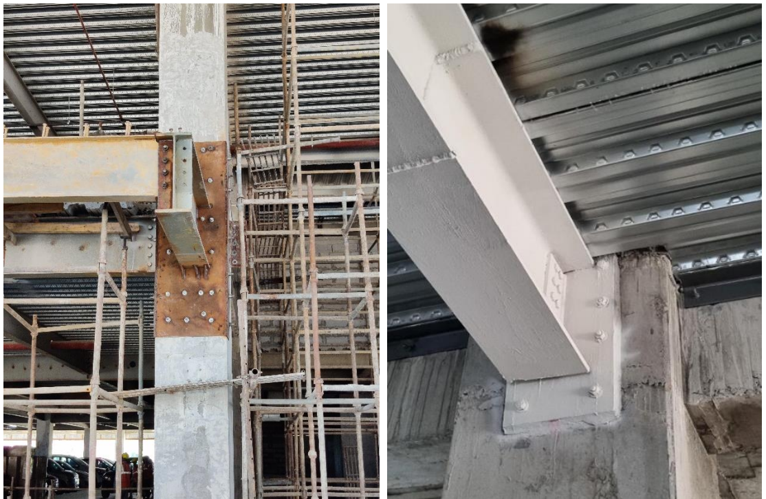
Fig. 1.1: Critical anchor arrangements at jobsite
