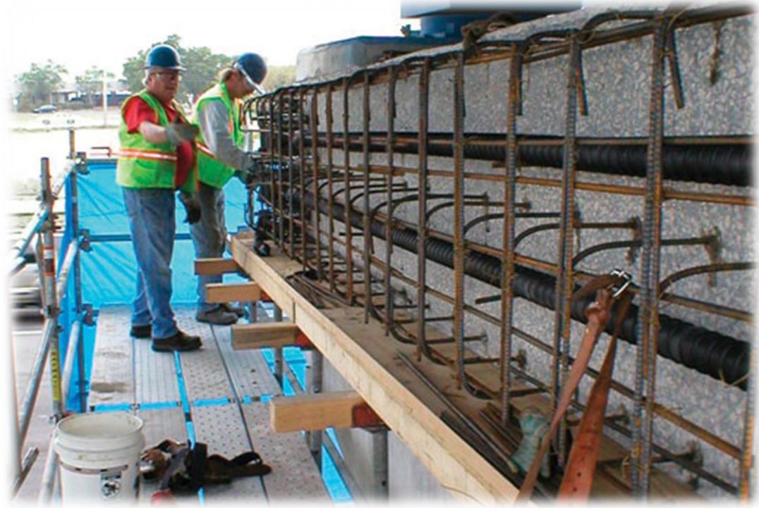
Beam strengthening
