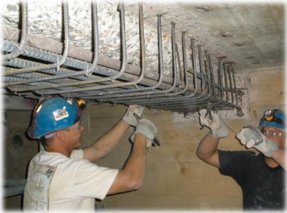
Beam strengthening
