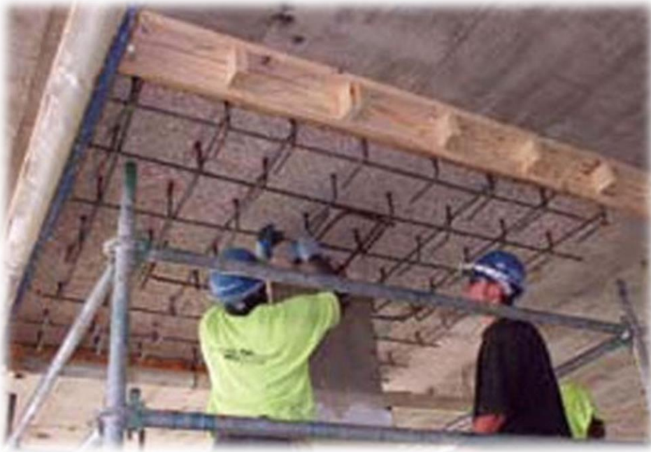
Slab strengthening
